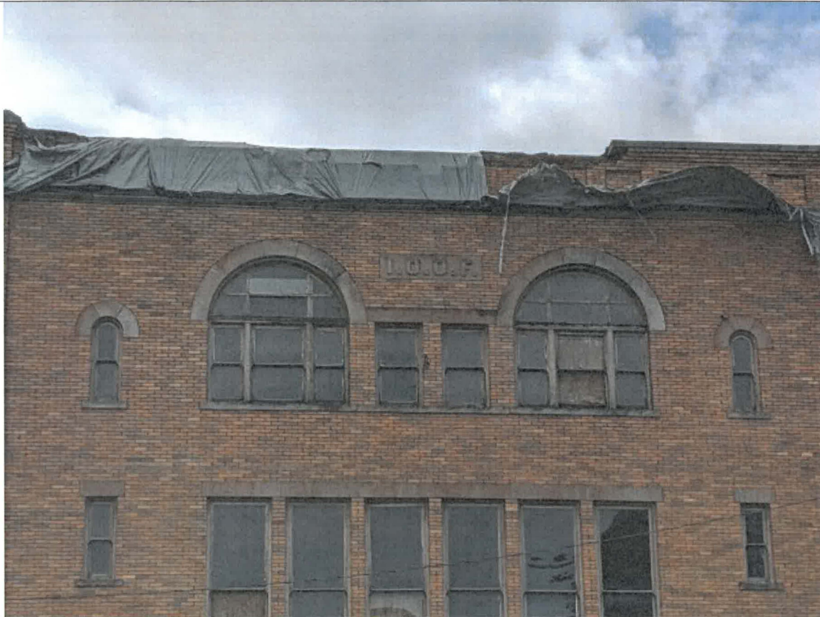
Façade of the I.O.O.F. portion of the building, showing parapet under the black plastic, facing south-southwest
