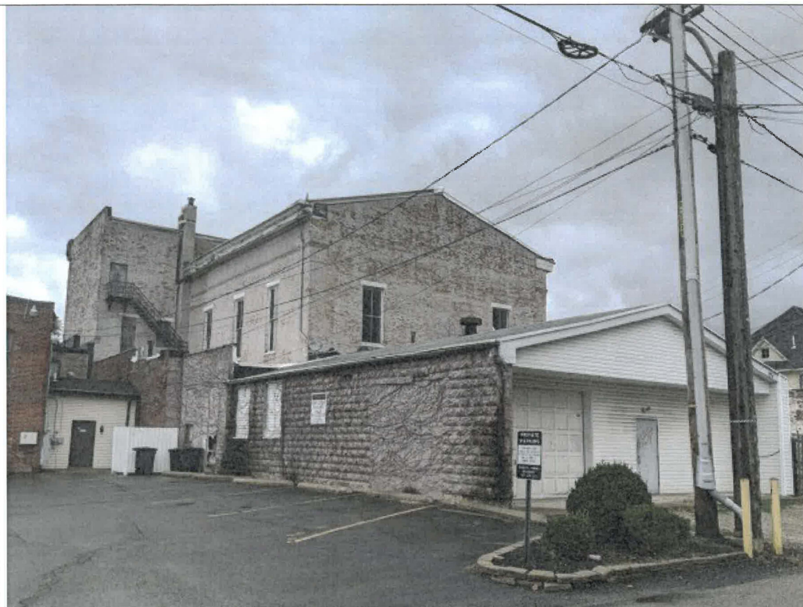
Back of building, showing portion of the original county courthouse, facing northeast.
