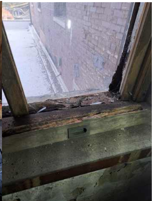
Rail of window in SE elevation (bottom of window) has rotted off
